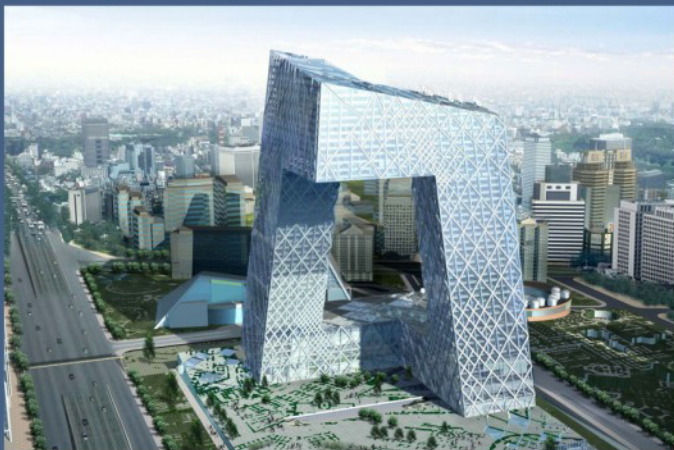
CCTV Headquarters, Beijing
