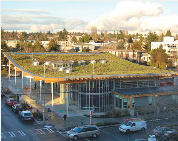
Ballard Library in Seattle, Washington captures and temporarily stores rain water to reduce flooding of sanitary and storm water sewers. Needless to say it also provides excellent thermal protection to the building.
